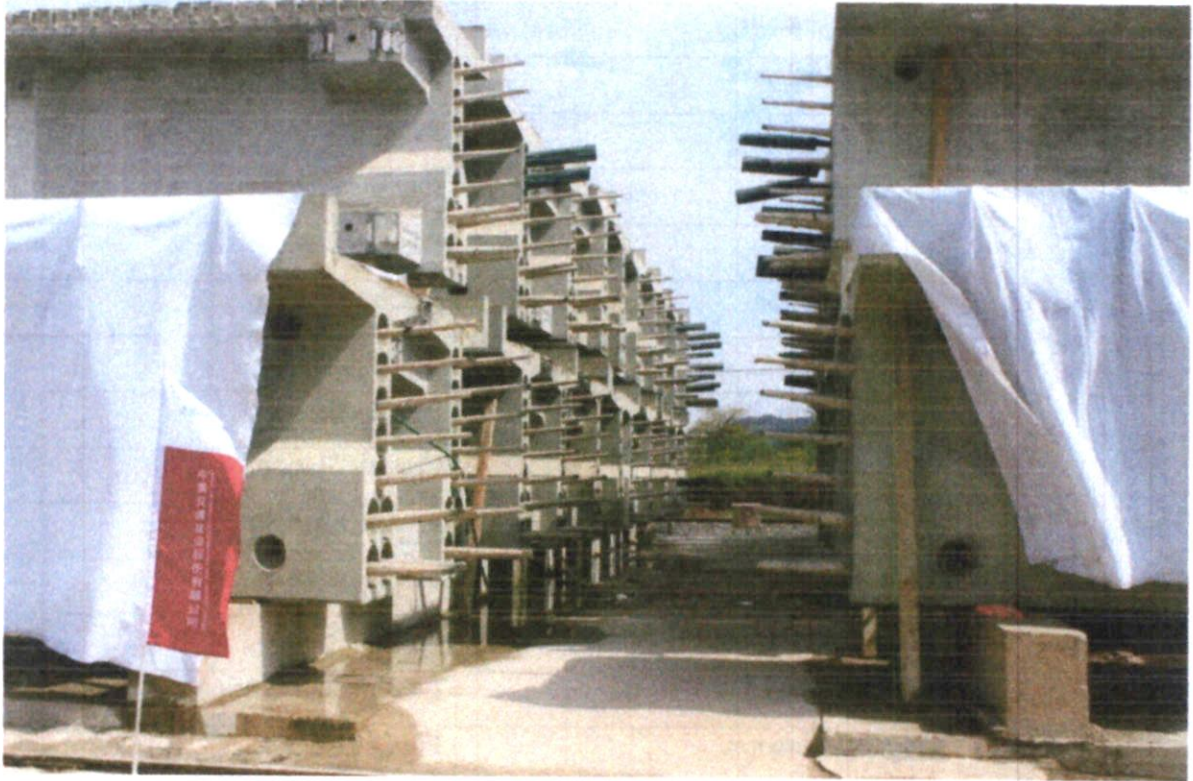
Picture 7: T-Beams ready for transportation to site
