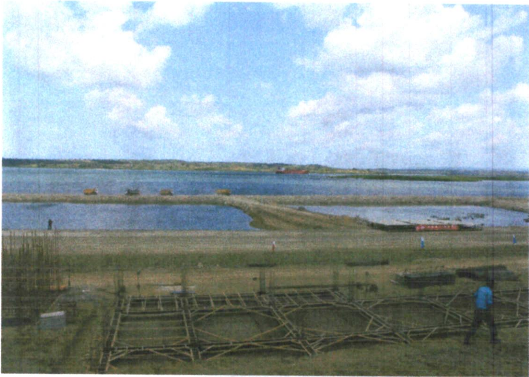
Picture 13: Ongoing construction site at Port Reitz Station in Mombasa
