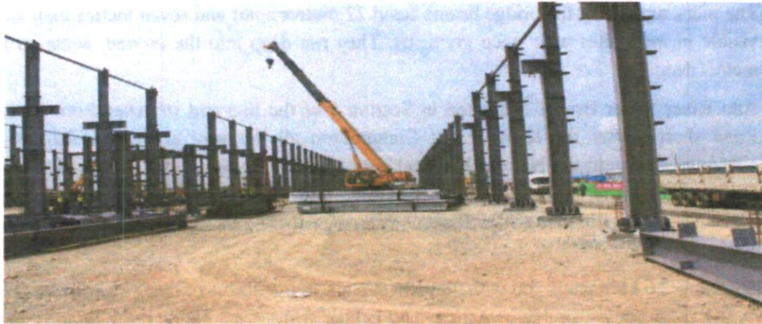
Picture 2: Ongoing construction Work at Nairobi SGR Terminus construction site
