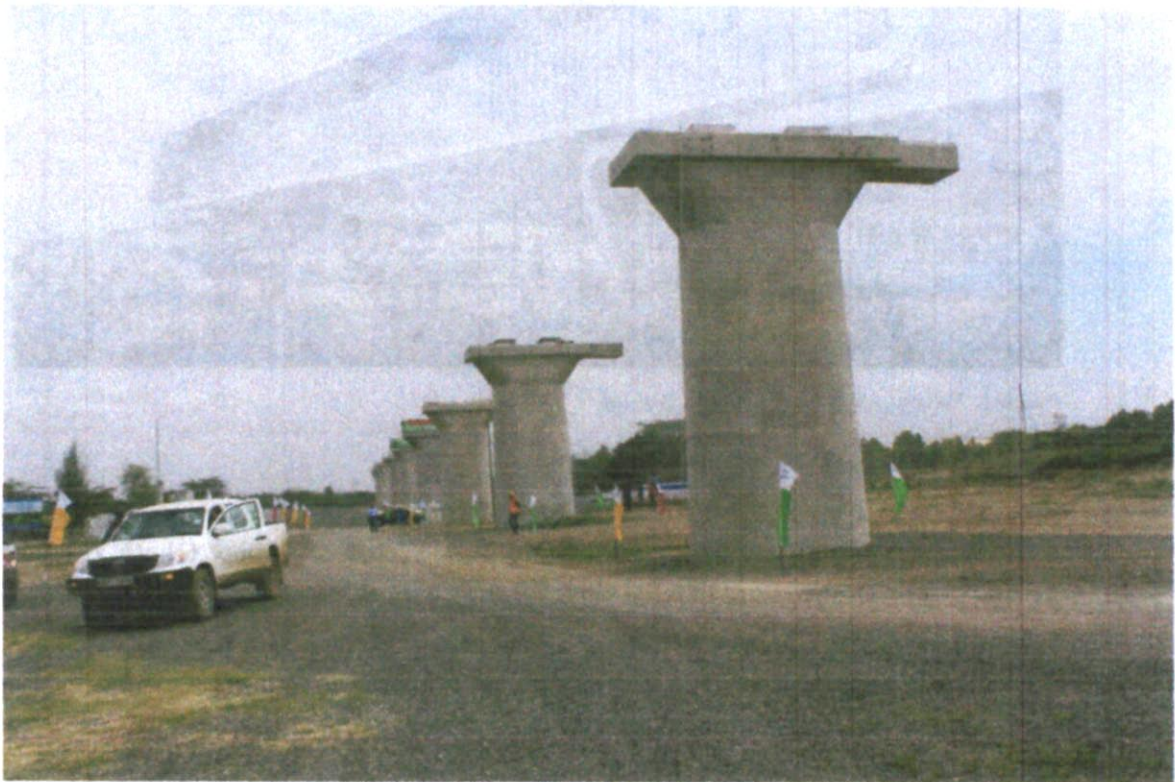
Picture 4: Construction of Athi River Super Bridge
