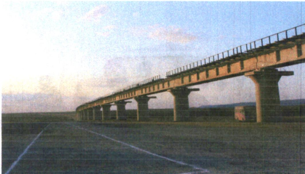
Picture 9: View of Tsavo Super Bridge
