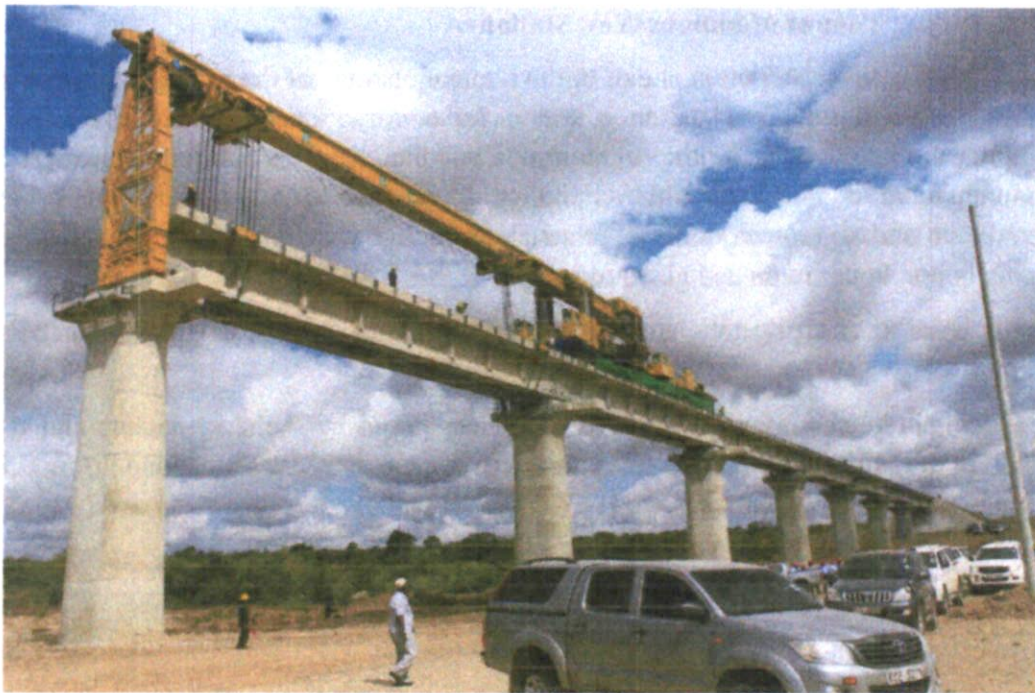
Picture 10: Ongoing construction work at Taru Super Bridge
