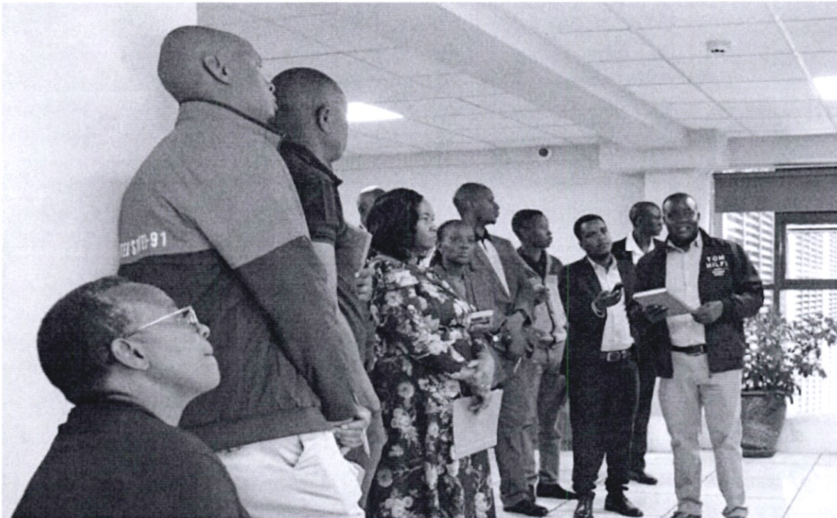
Figure 1. KENHA team undertaking the Committee through the operations of the data centre.
