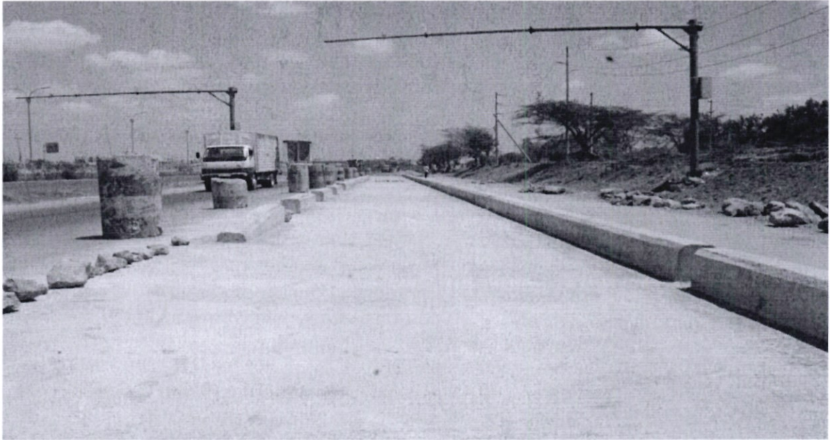
Figure 3. High speed weighing lane at Mlolongo Weighbridge
