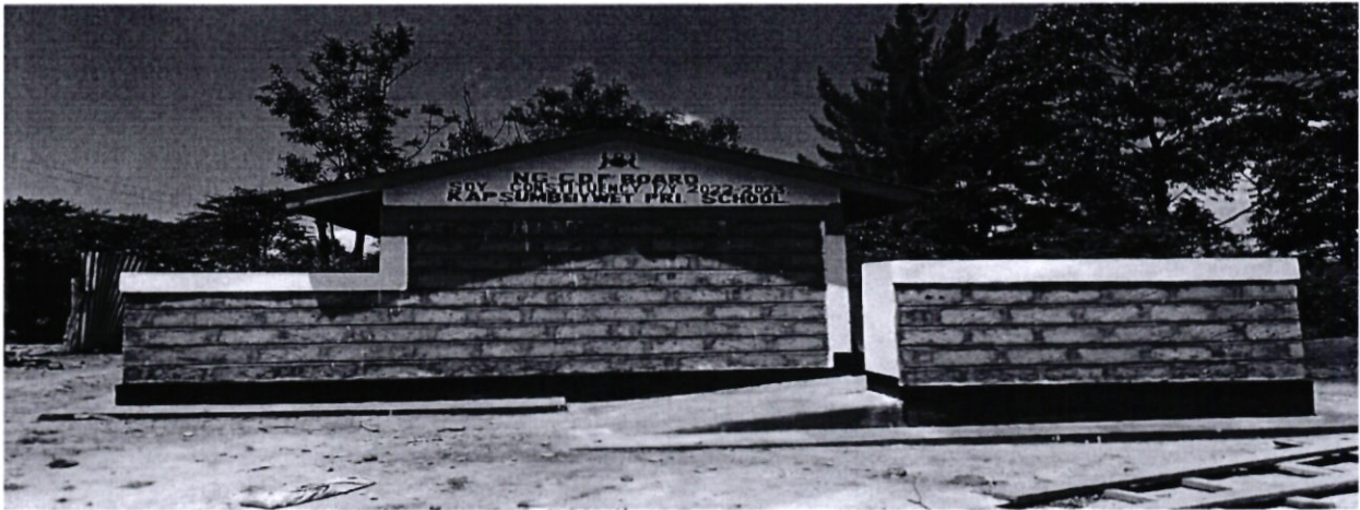
Kapsumbeiywet Primary School Construction of four door Pit Latrine
