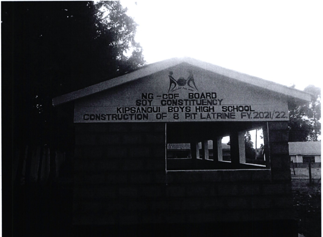
Kipsangui Boys High school Construction of eight door pit latrine
