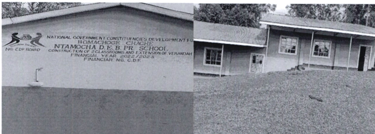
Photo: Construction of 2 Classrooms and Extension of Verandah at Ntamocha Pri. School.
