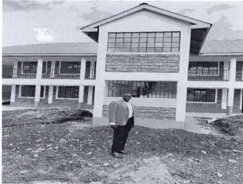
Photo: Bomachoge Chache KMTC Project, Ongoing Phase II
