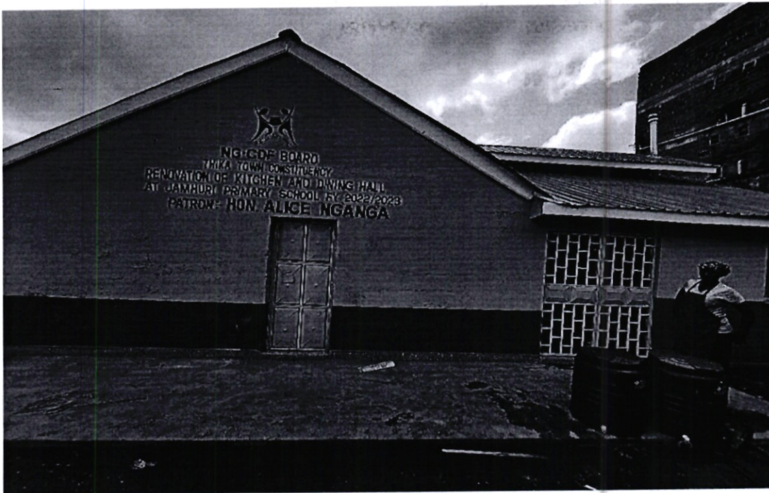
Renovation of Kitchen at Jamhuri Primary School
