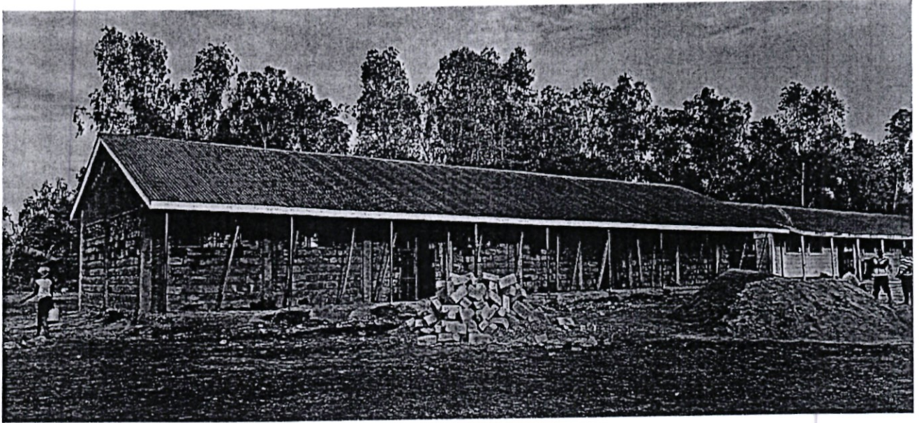
MAREGA PRIMARY SCHOOL – ONGOING CONSTRUCTION OF THREE CLASSROOM – 2022/2023
